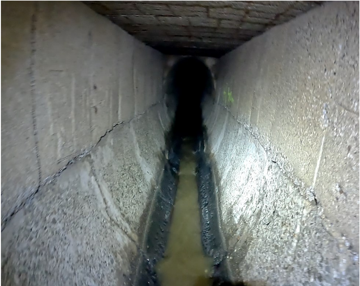
Fig. 1.1: egg-shape profile W:H = 1100:1850 mm; straight section in front and normal section in the back
